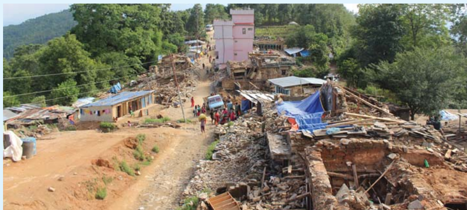
A devastating view of Nawalpur, Sindhupalchok
