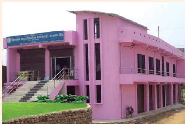
Building of Kisan Bahuudeshiya Sahakari Sanstha Ltd.
